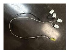
Reconnect the existing half of the yellow disconnect from the ceiling to the new retrofit disconnect.
